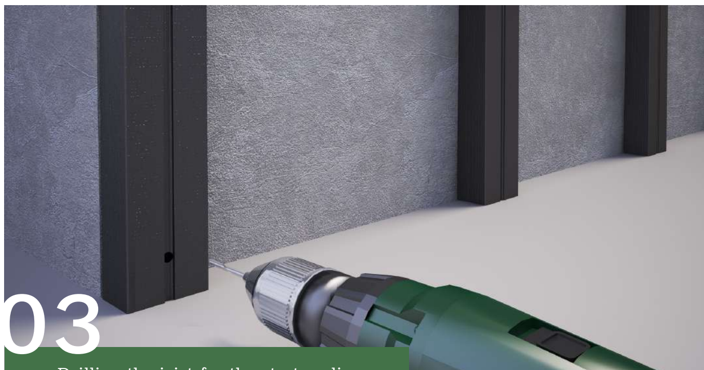
Drilling the joist for the starter clip
