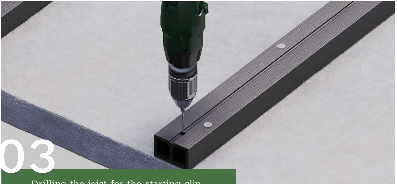
Drilling the joist for the starting clip
